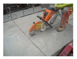
Figure 10: Cutting Walls (a) Horizontally and (b) Vertically
