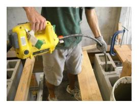
Figure 8: (a) Grout Funnel Leading into One Grout Column and (b) Mechanical Vibration
