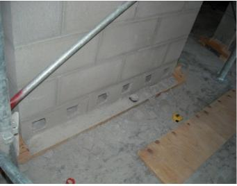
Figure 7: (a) Wall Elevation and (b) Location of Cleanouts at Bottom of Wall
