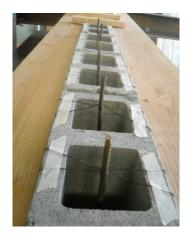
Figure 6: Wall Construction (a) Horizonal Steel Placement and (b) Vertical Steel Placement
