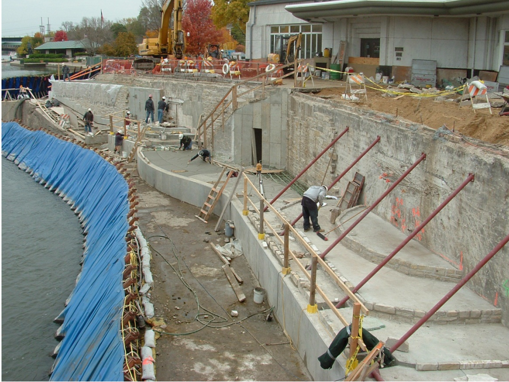
Figure 8: Overall View of Construction
