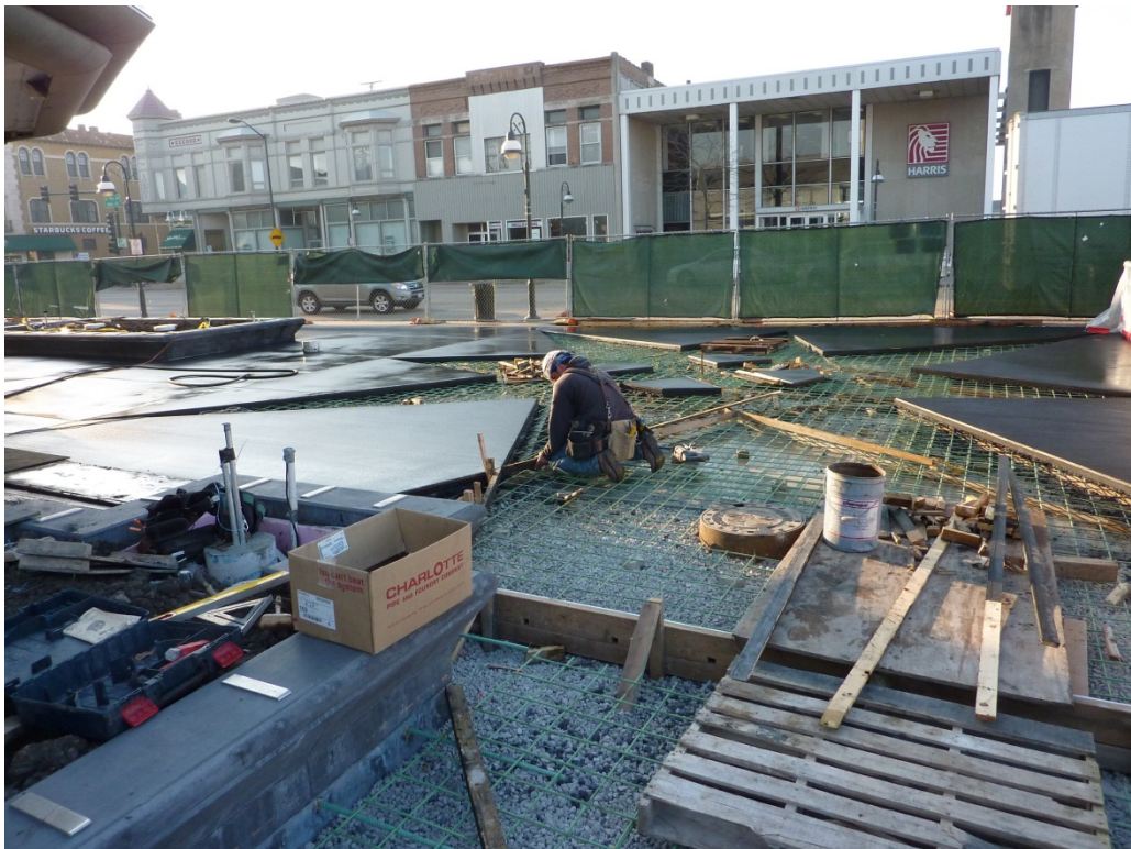
Figure 9: Installation of Integrally Colored Concrete
