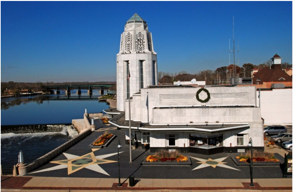
Figure 10: View of Plaza from South Following Completion of Reconstruction
