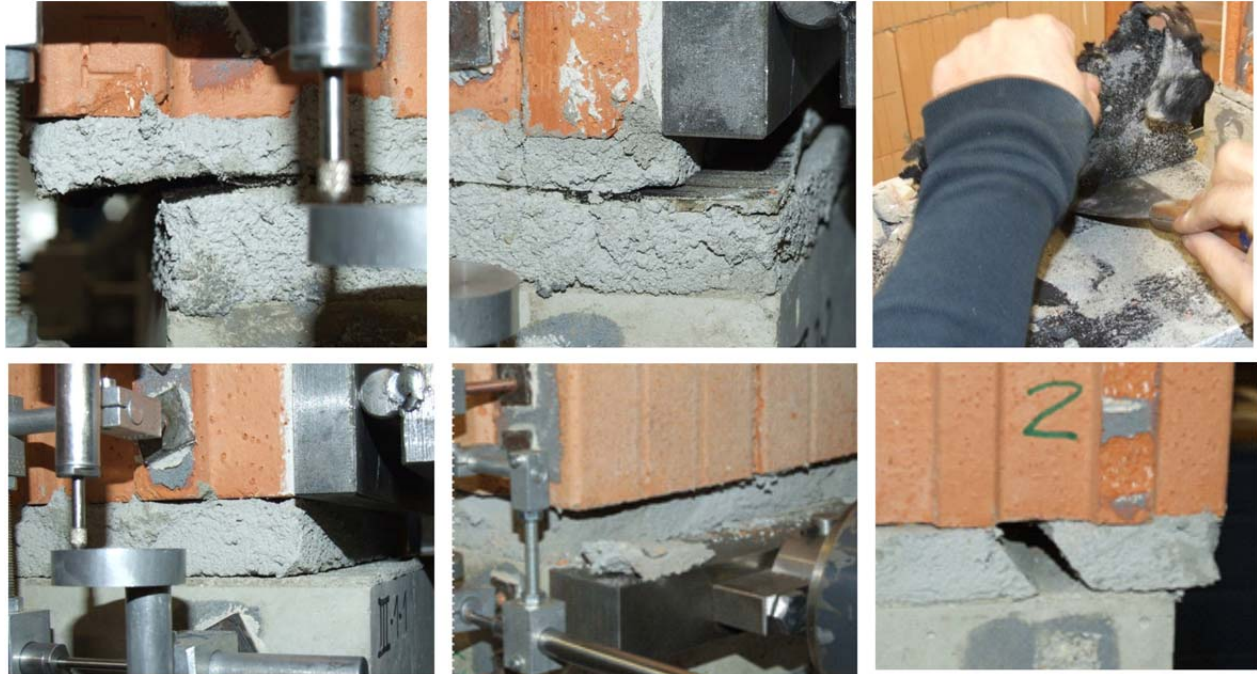
Figure 5: Typical Failure Cases of the Bond in the Bed-Joint:
