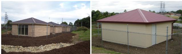
(a) Brick Veneer and Cavity Brick Modules Figure 3: Housing Test Modules
