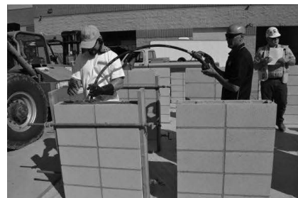
Figure 5: Consolidating Grout
