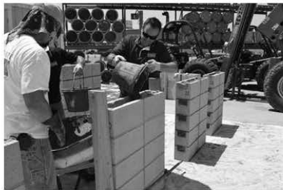
Figure 4: Bucketing Grout into Sample Panel
