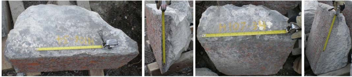
Figure 2: Comparison of two face stones removed from the north wall
