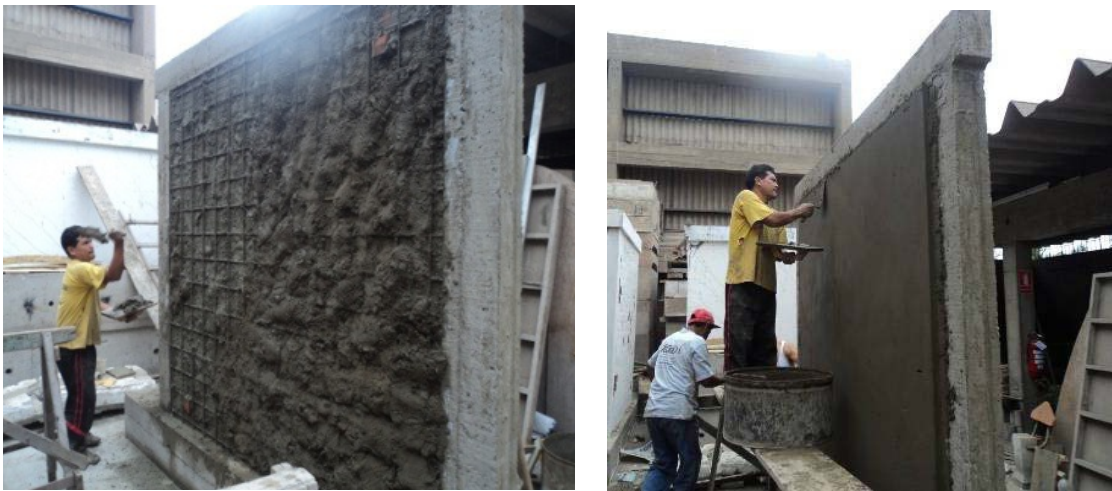
Figure 8: Cover of wire meshes in W2, done in two steps
