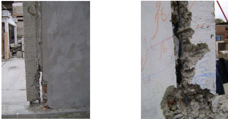
Figure 11: Wall W2 inspection after the tests
