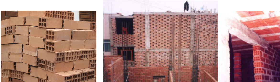
Figure 1: Horizontally hollow bricks used in self-constructions for bearing walls in Peru
