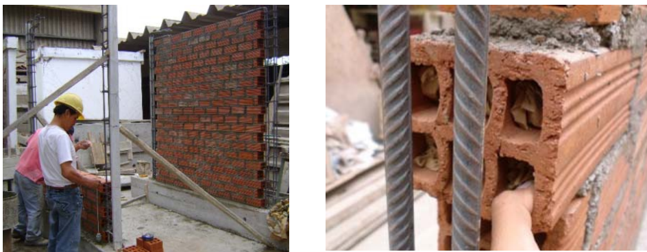
Figure 6: Construction of walls W1 and W2.
