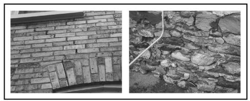
Photo 12: (Left) Cracks caused by deterioration of inner core rubble. Photo 13: (Right) Condition of below grade foundation wall.
