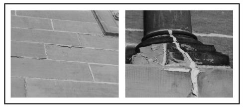
Photos 2 & 3: Examples of damage caused by the deterioration of inner core rubble
