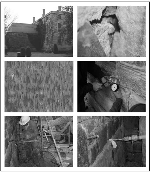
Photo 14 (Top Left) Former County of Peel Jail - the grouted courtyard wall is to its left. Photo 15 (Top Right) Example of inner core rubble deterioration after removal of stone masonry unit. Figure 1 (Middle Left) Computerized contour image produced by GPR - The darker areas represent solid masonry. Photo 16 (Middle Left) Pullout testing a masonry tie. Photo 17: (Bottom Left) Pumping cellular grout through an injection port. Photo 18 (Bottom Right) Contact is made between ports.
