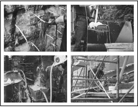
Photos 8: (Top Left) Flushing the core with warm water. Photo 9: (Top Right) Pumping foam into mortar mixer. Photo 10 (Bottom Left) Transferring cellular grout to pump hopper. Photo 11: (Bottom Right) Injecting cellular grout into inner core rubble.
