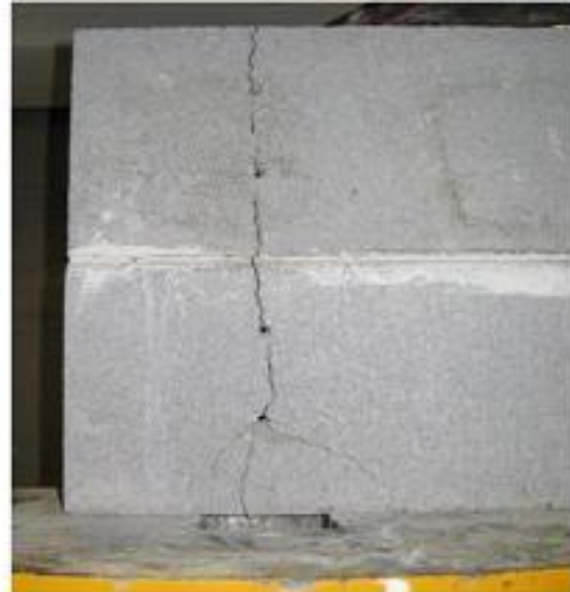
b) Failure of block along line of screws
