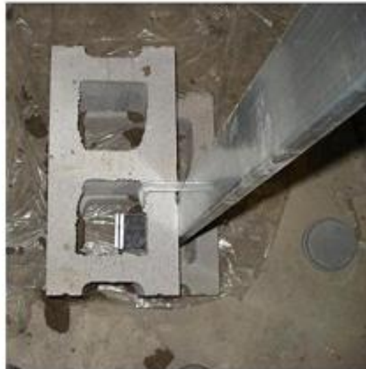
d) Tie anchorage in ashlar block before grouting
