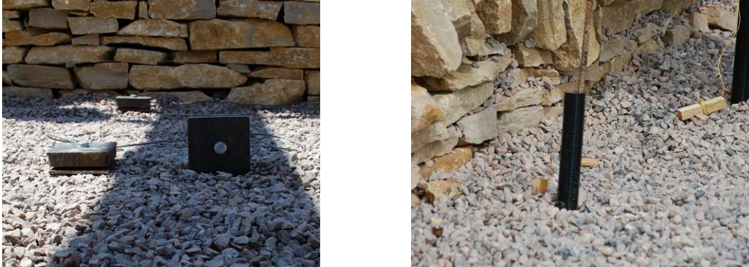
Figure 4: Instrumentation: a) backfill load cells; b) inclinometer tubes
