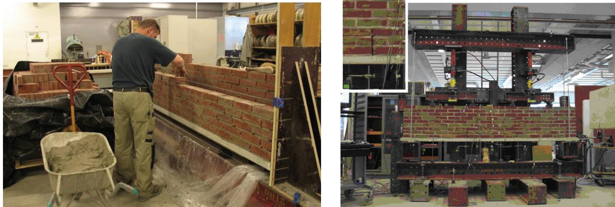
Figure 5: a) Building the test walls, in the TU/E laboratory. b) Test set up roller support with, in detail, open header joints above the lintel
