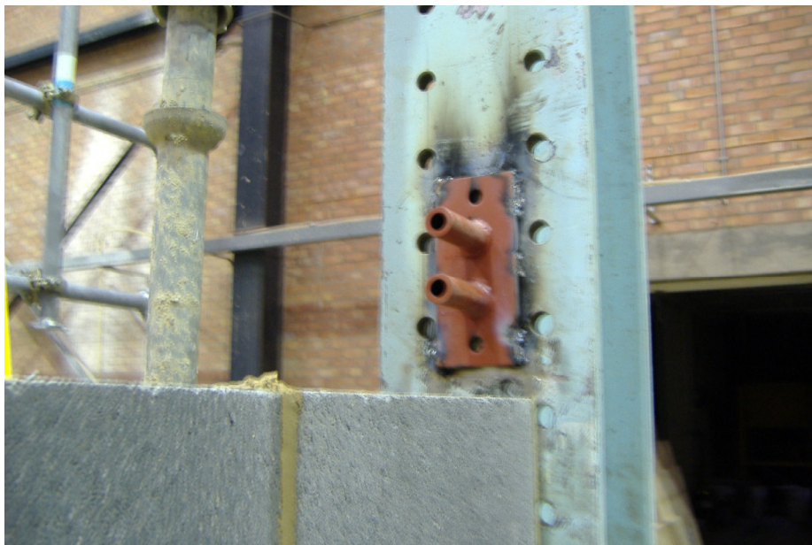
Figure 2: Cleat Welded to Steel Column
