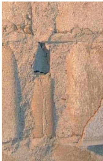
a) Partial grouting of head joint cell
