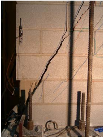
a) Wall 1, East Toe
