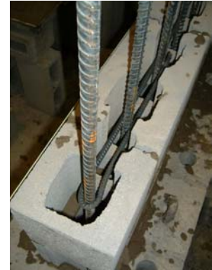
d) Knock-out web blocks with vertical and horizontal reinforcement
