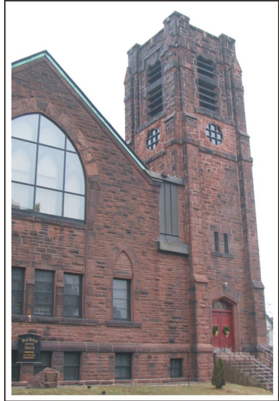
Figure 26 - The restored and stabilized bell tower
