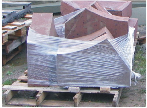
Figure 21 - Fabricated voussoir stone units ready for shipment to the church.
