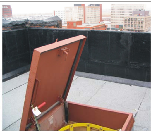
Figure 23 - Waterproofed new deck with watertight hatch.
