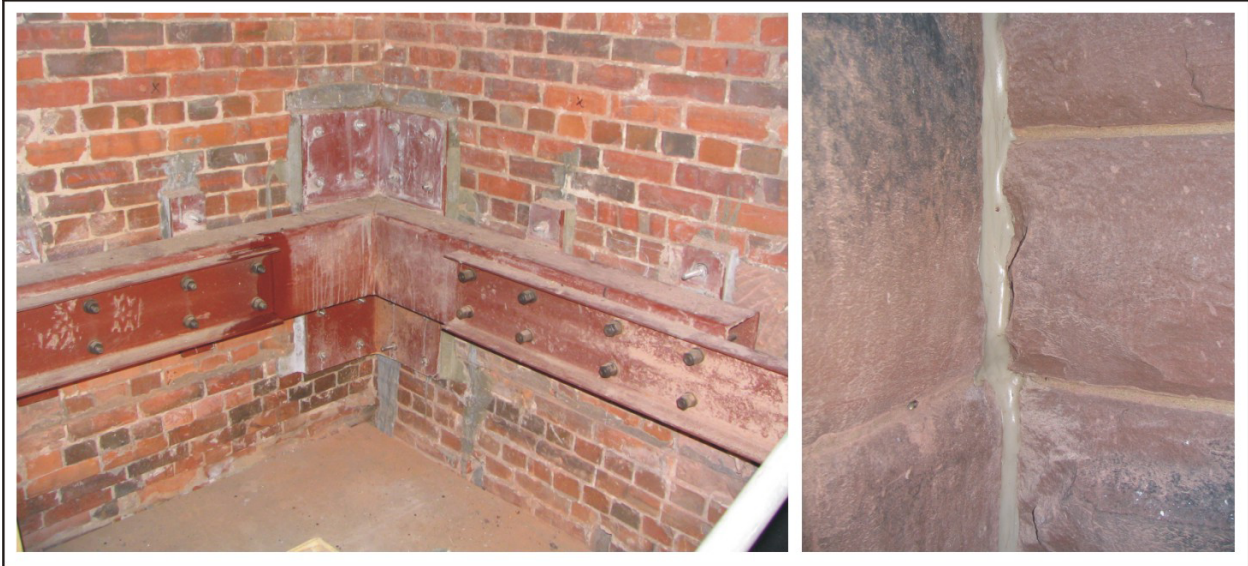
Figure 12 - Sliding beam and anchorage arrangement.
