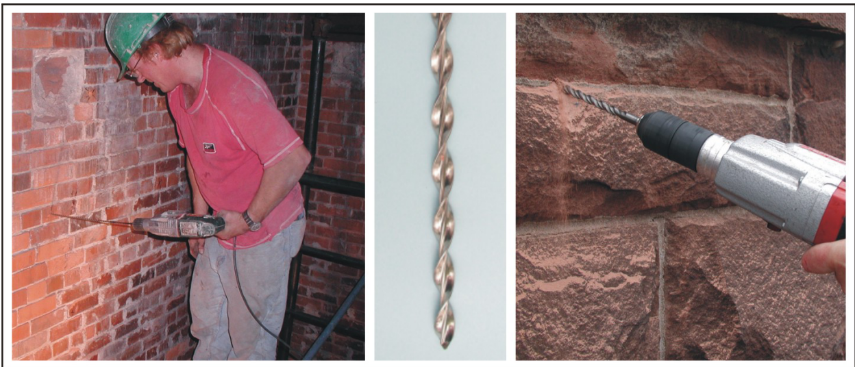
Figure 14 - Installing ties from interior.
