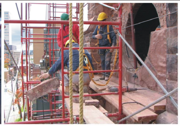
Figure 18 - Lowering one of the voussoir stones to ground level.
