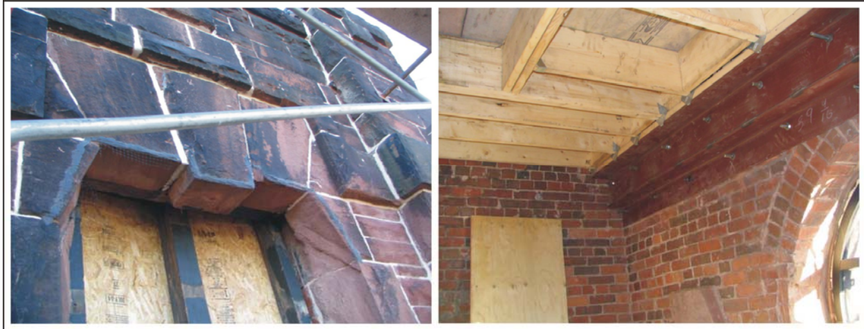
Figure 24 - The dislodged keystones were repositioned.
