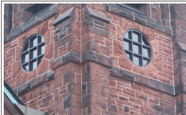
Figure 22 - New round windows installed within the reconstructed masonry.
