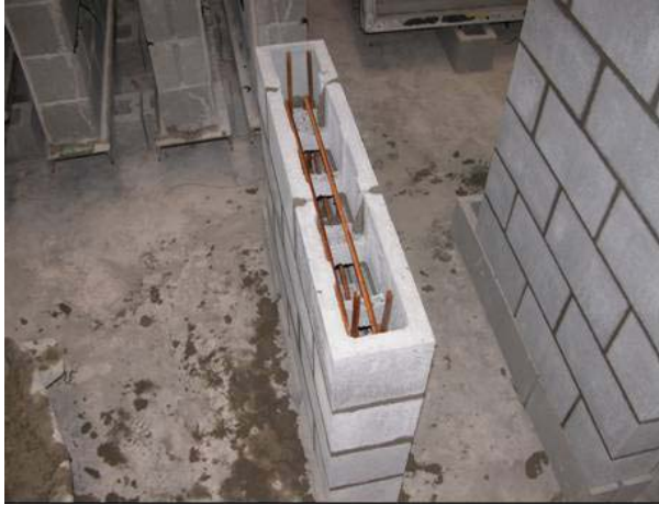
Figure 2 – Placement of Confinement Reinforcement
