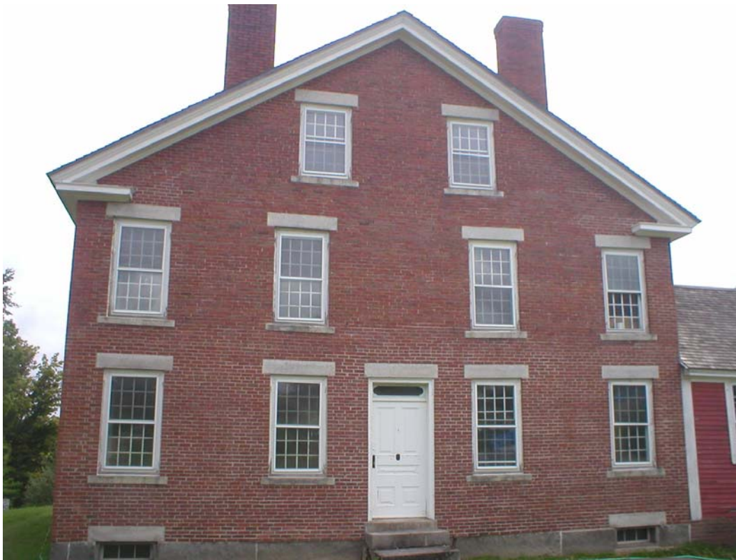
Figure 15 – West Wall after Restoration
