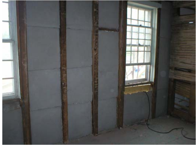
Figure 11 – Brick Nogging with Parging Installed
