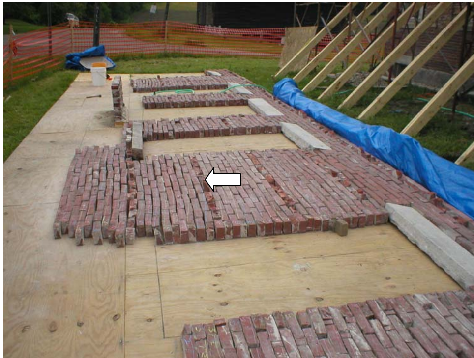
Figure 13 – West Wall Exterior Veneer
