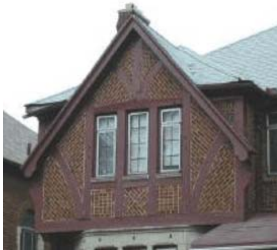
Figure 1 – Brick Nogging on a Residence
