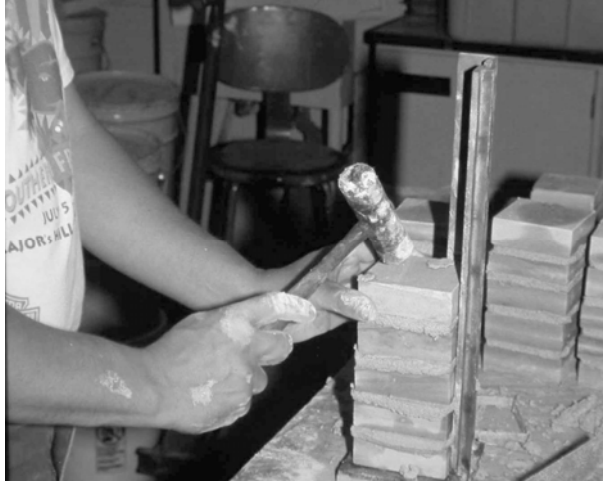
Figure 1 – Mason Building Masonry Prisms (phase 1)
